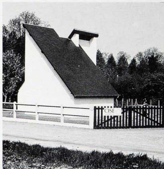
Rots (14) . Station de pompage AEP
